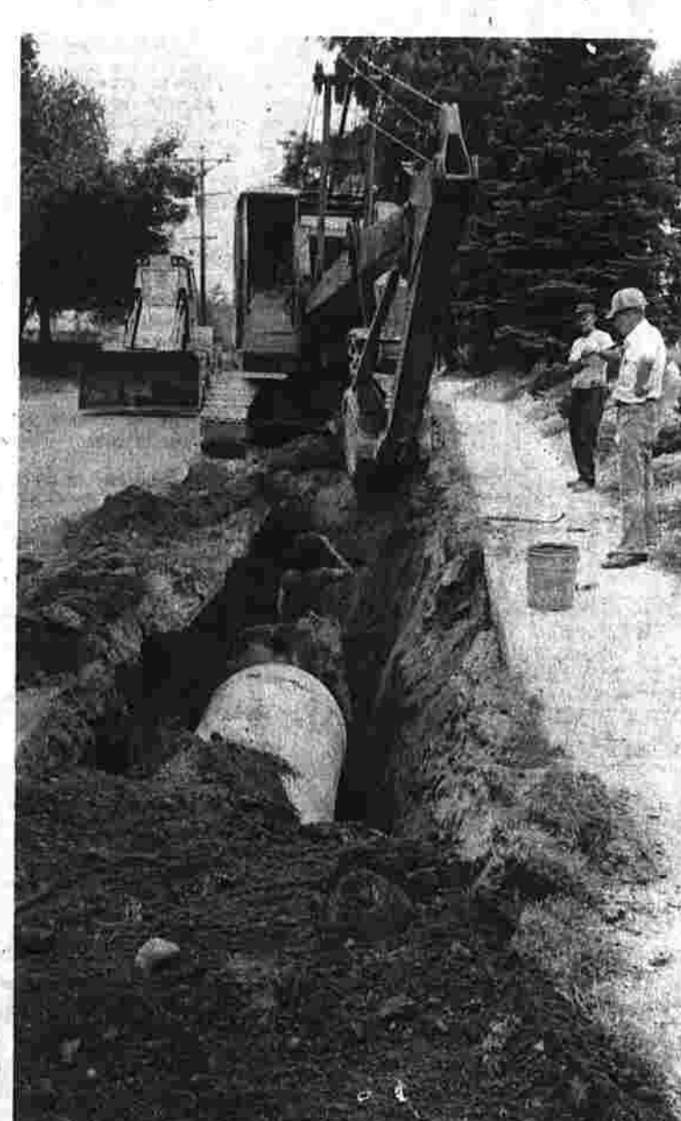
Work is proceeding on the west side of Keeney St., from Folly Brook south to Linwood Dr., on the installation of sanitary sewers. This trench is almost exactly opposite Keeney St. School. In it is Al Otis, who works for A. Dzen Co. of Manchester, contractors for the project. On the sidewalk, in the foreground, is George Blake, the town's construction inspector. Beyond him is Hap Dodd, an A. Dzen employee. Sanitary sewers already have been installed in other sections of Keeney St., south of this project. Tonight, the Board of Directors will consider a $77,000 appropriation (to be financed from assessments against abutting property owners) for Keeney St. sanitary sewers from Hackmatack St. to Folly Brook. (Herald photo by Pinto)
